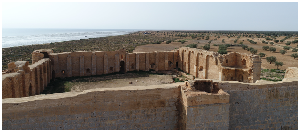
Figure 10: Restoration of the top of the mud-walls with white mortar
